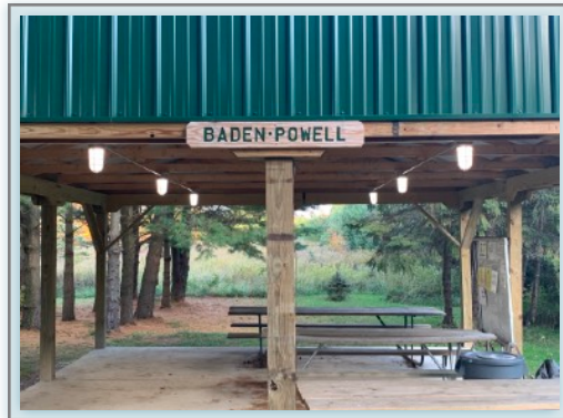
Solar power, lights, and concrete padding for Baden Powell Shelter
