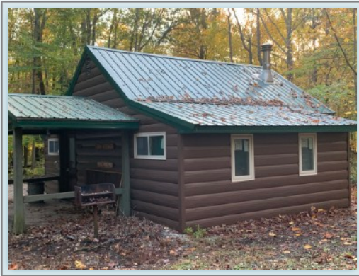
New windows for the renovated Lorain Exchange Cabin
